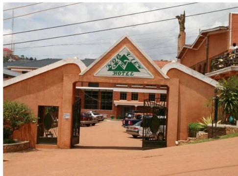
Hotel Main Entrance
